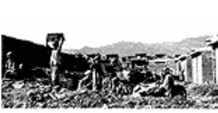
Fig. 35. First community of lower income housing under construction
