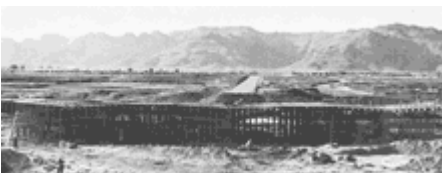
Fig. 22. The intersection of the Islamabad and Murree highways under construction
