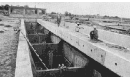
Fig. 21. Sewage aeration tank in Islamabad, during construction
