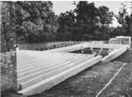
Fig. 20. Water softening installations at the Nurpur spring
