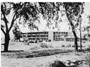
The Student Hostels under construction
