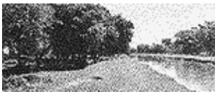
Detail of the Site
