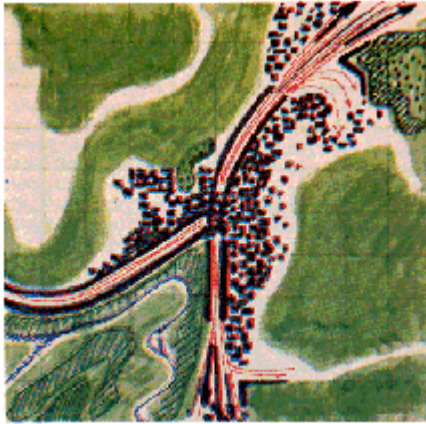
Fig. 12. Open the road for the explosion
